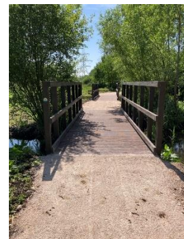
New bridges are made from steel and recycled plastic, with long life spans in damp environments
