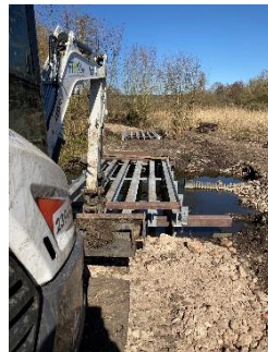
New bridges are made from steel and recycled plastic, with long life spans in damp environments
