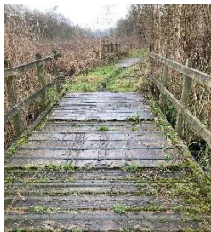
Old wooden bridges were rotting from the wet conditions
