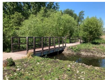
New bridges are made from steel and recycled plastic, with long life spans in damp environments
