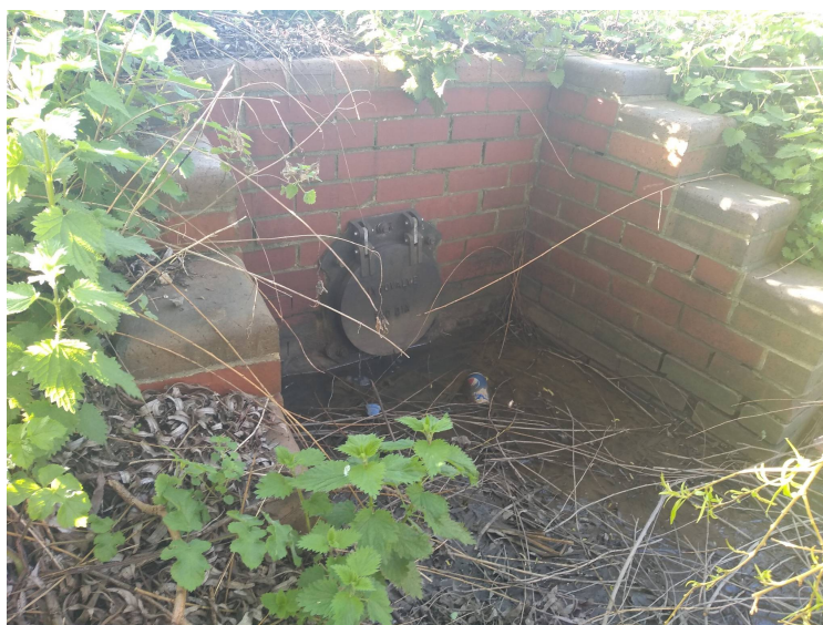
Figure 14. Example of an outfall pipe in the Colne Valley
