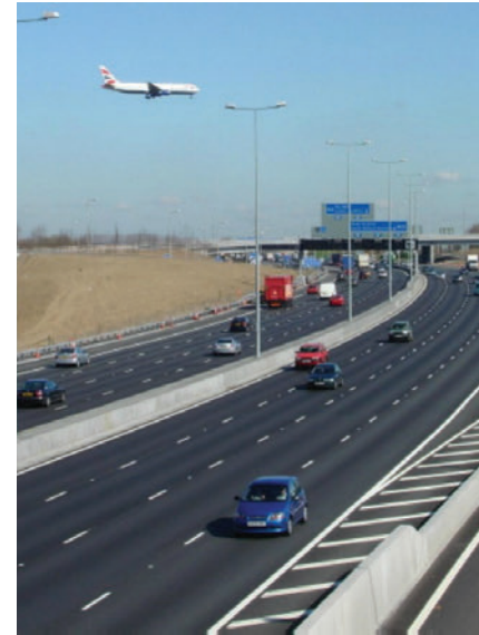
Motorway infrastructure and Heathrow airport dominate parts of the valleys
