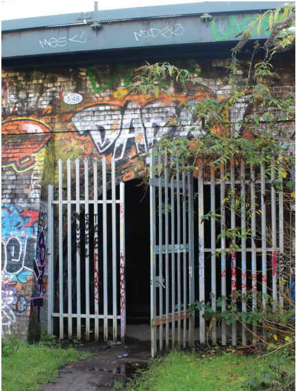
Railway underpass / Cranewalk
