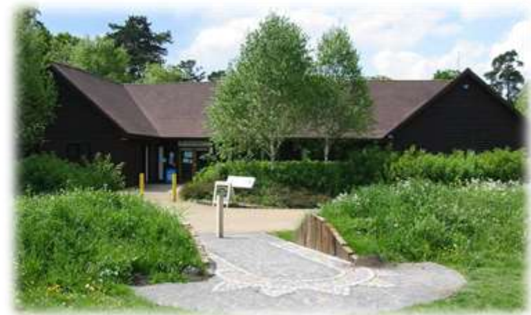
Colne Valley Visitor Centre on a Buckinghamshire CC landholding – Groundwork South
